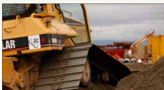
AIC began work on Kotzebue's Front Street summer 2010.
