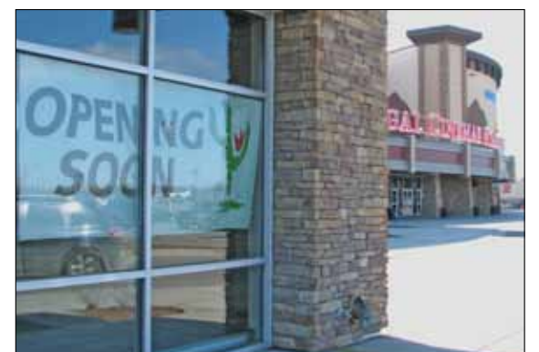
Qdoba is constructing a new restaurant adjacent to the Regal Tikahtnu Stadium 16 IMAX theatre at Tikahtnu Commons, Alaska's largest shopping destination.
