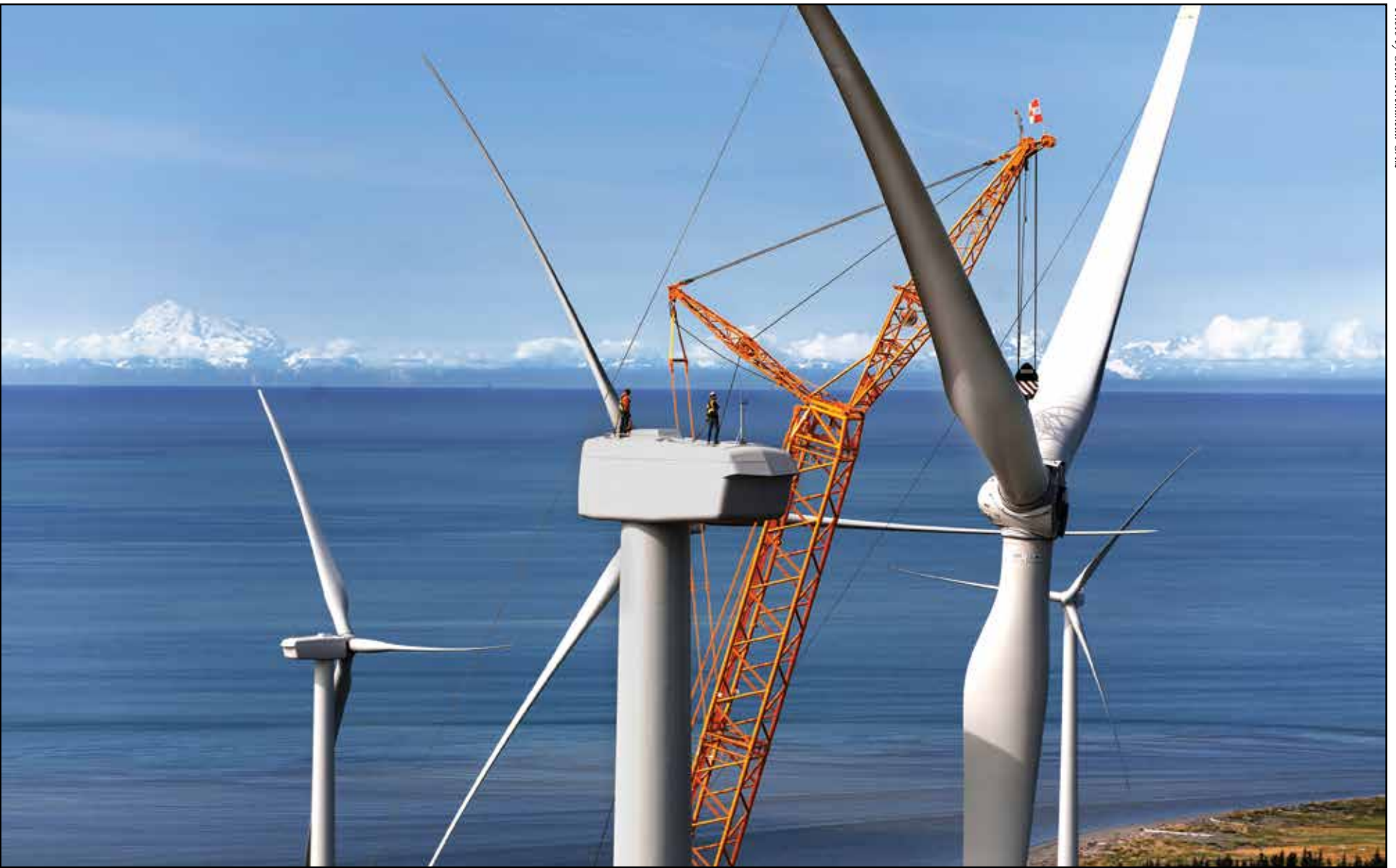
Workers stand on top of the turbines' 262-foot-tall hubs with safety straps and harnesses to direct each turbine rotor assembled with the only 660-ton crane in Alaska.
