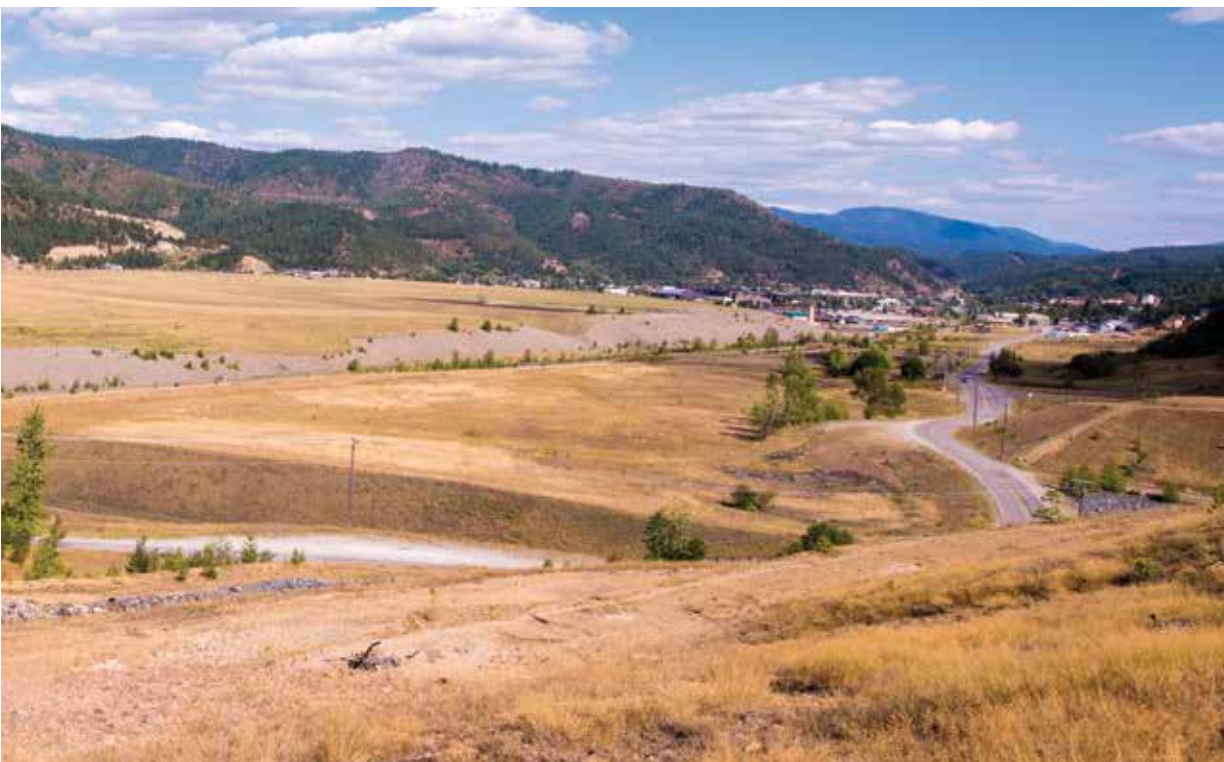
› The city of Kellogg, Idaho, (in the distance) and the massive pile of mine tailings, known as the Central Impoundment Area, from the Bunker Hill Mine. Photo by Jason Moore.
