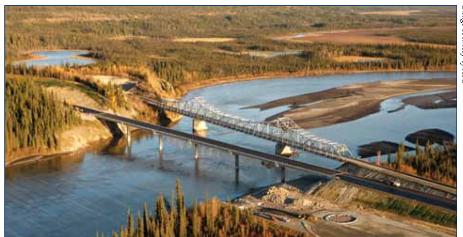
The new Tanana River Bridge stretches a half-mile across the Tanana River near Tok and replaces a bridge built during World War II.
