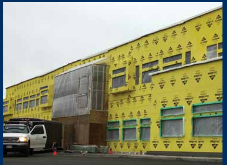
Construction at 11500 C Street progresses on schedule into the winter season. Photo taken on Oct. 25, 2010.
