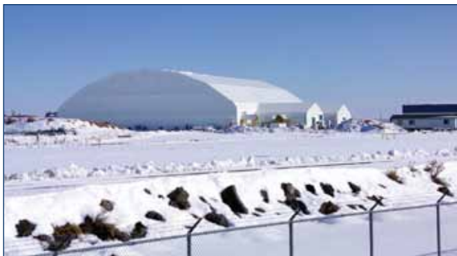
North Wind Services begins construction on a hazardous waste retrieval structure in Idaho.
