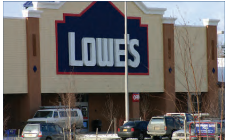
Lowe's new home improvement store at Tikahtnu Commons opened on April 1. The national retailer is among the many shops and stores opening at the Northeast Anchorage retail center throughout 2009 and 2010.
