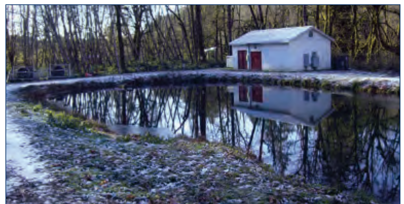
ANC Research & Development LLC was recently awarded a contract to restore this effluent pond at the Abernathy Fish Technology Center in Longview, Wash.
