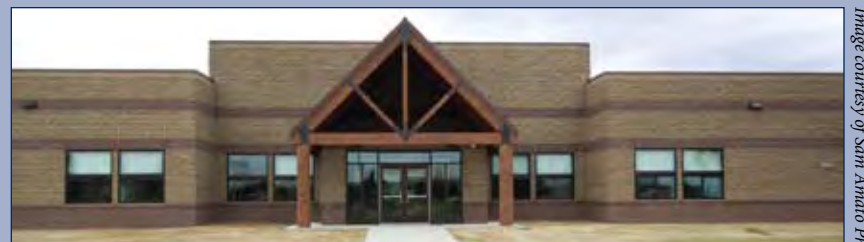
Weldin Construction recently won an award from the U.S. Air Force for its work on the Professional Military Education Center at Elmendorf Air Force base.
