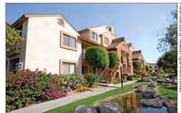
Photo courtesy of Weidner Apartment Homes
