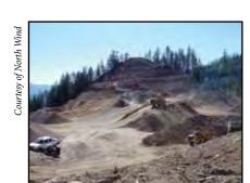
A waste consolidation area is being built by North Wind to properly store contaminated soils produced by silver mining operations.
