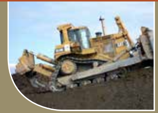
CIRI sells construction subsidiary | 04
