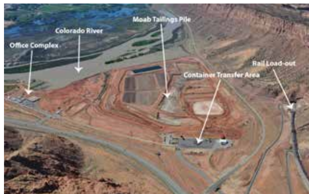
▶ A bird's-eye view of the Moab UMTRA project.
