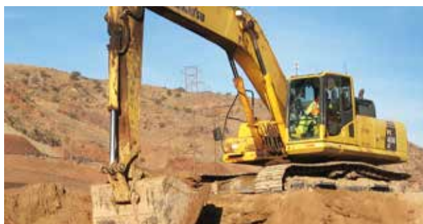
An excavator removes contaminants at a project site.
