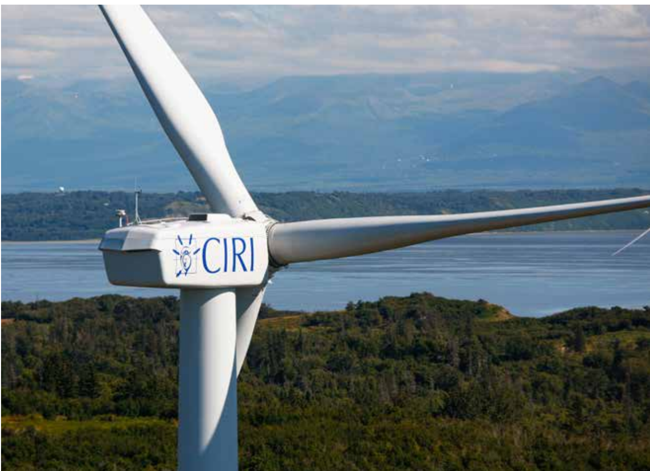
➤ In January, the Fire Island Wind Project achieved its best-ever month of production: 7,260 megawatt hours and 99 percent availability. Photo by Judy Patrick.
