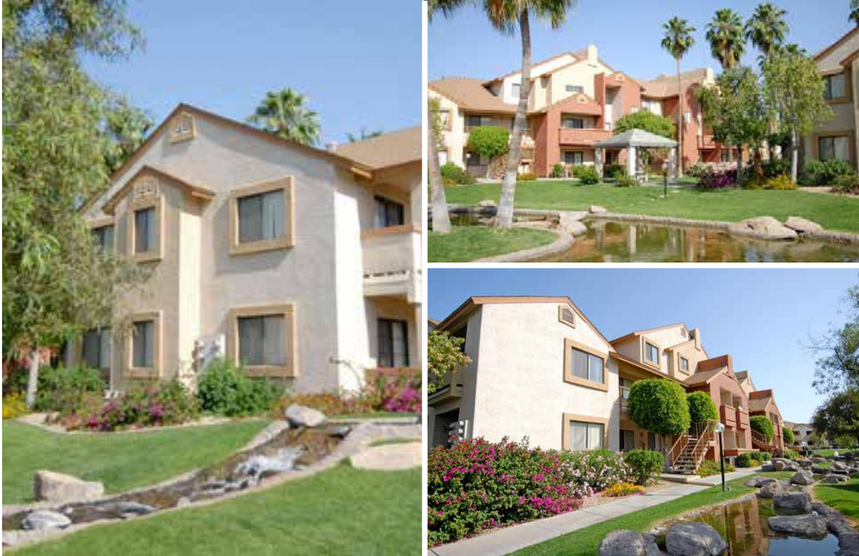
› The 768-unit Red Mountain Villas apartment complex features timeless architectural design and an array of luxurious community amenities.
