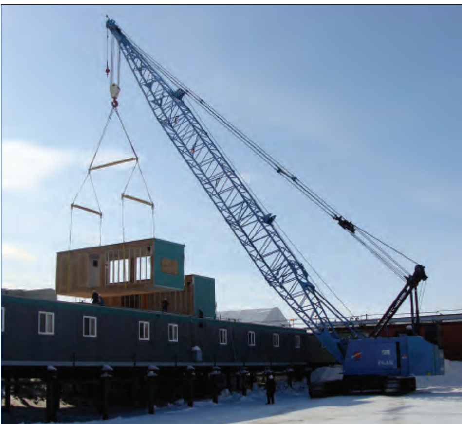
Peak has a large and versatile fleet of heavy cranes ranging from 50 to 300 tons that support a variety of oilfield development and maintenance activities.
