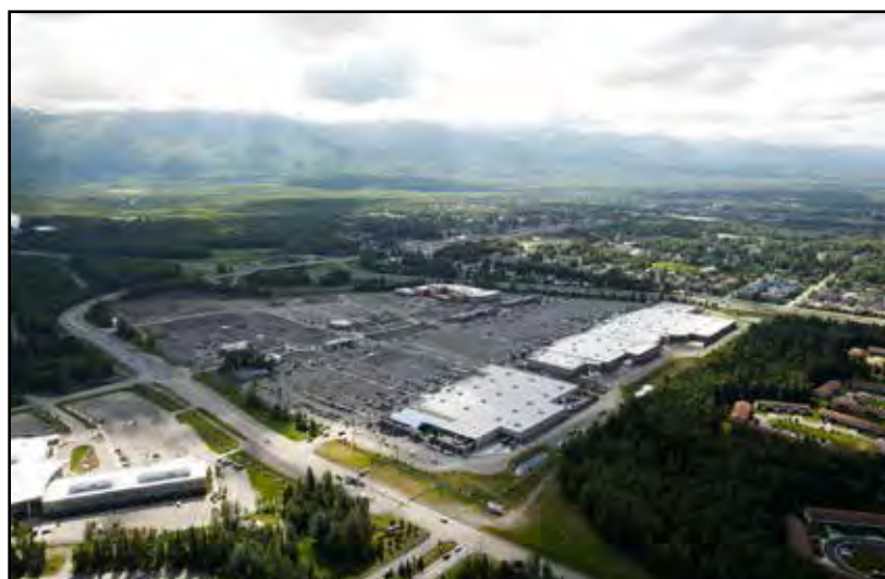
An aerial view of Tikahtnu Commons, summer 2012.
