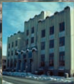
Fairbanks Post Office, acquired as federal surplus property in 1979, was converted to office condominiums.
