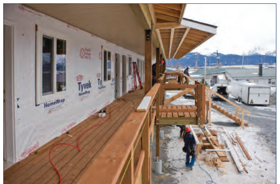
Local workers build Kenai Fjords Tours' new bunkhouse in Seward, Alaska.
